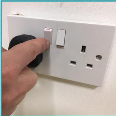
Fully unwind the supply cord and plug in to a convenient socket outlet.
